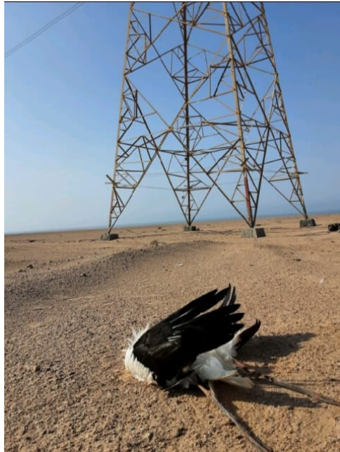
Figure 1 Dead White Stork under the El Tor - Sharm El Sheikh OHTL. August 2021 (photo NCE).
