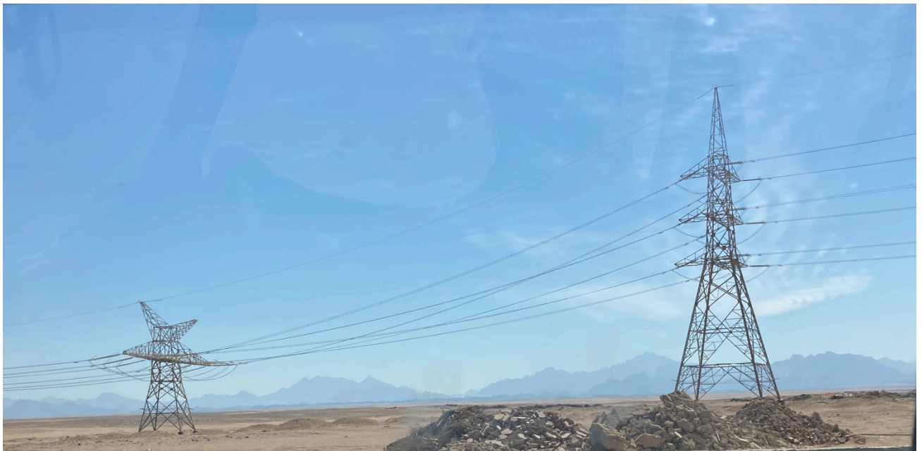
Figure 14. Transfer from the “normal” three tire transmission tower to a low lying tower with a single cross bar could reduce bird mortality, is considered a risk minimization technique. This example is implemented to the west of Hurghada, as well as, between Hurghada ad Gebel El Zeit, though other “normal” height power lines have been established in the same region.
